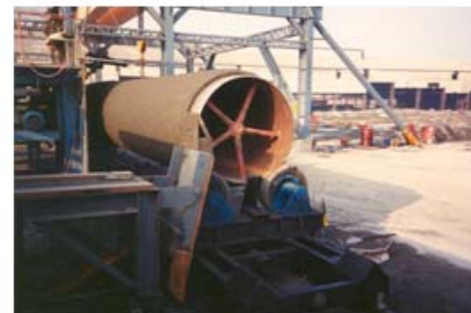
CONCRETKOTE® - CWC by IMPINGEMENT
